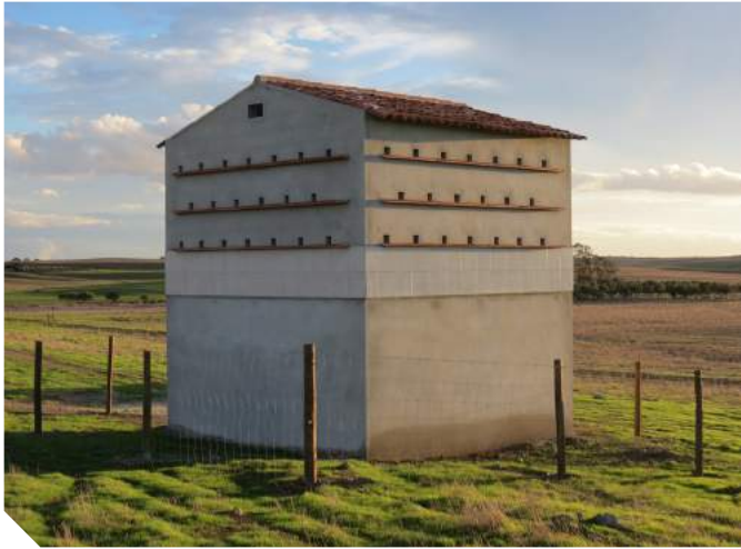
Breeding tower for Lesser Kestrel. This structure comprises 80 new nesting spots.
